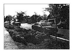
Bioswales are vegetated, mulched, or xeriscaped channels that provide treatment and retention as they move stormwater from one place to another. Vegetated swales slow, infiltrate, and filter stormwater flows. As linear features, vegetated swales are particularly suitable along streets and parking lots.
